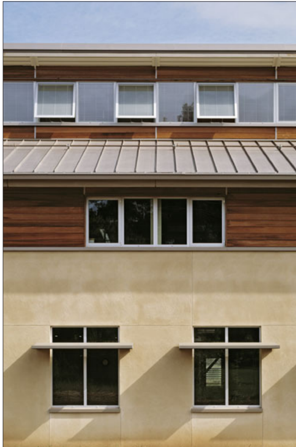
Pedestrian friendly and well modulated architectural facade incorporating ecologically-friendly elements including photovoltaics, light shelves and recycled materials
