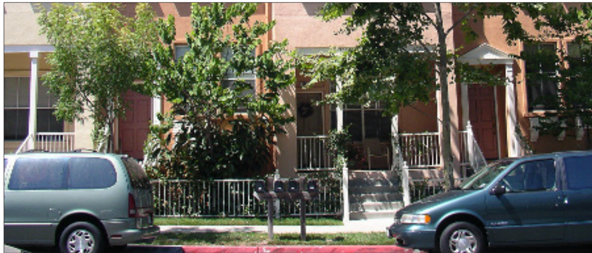
Well articulated building facades
