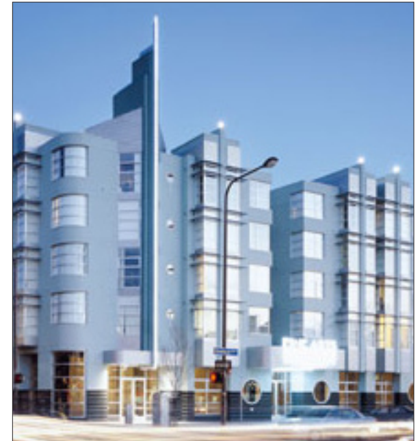
Creative lighting of buildings (1Avii-21)
