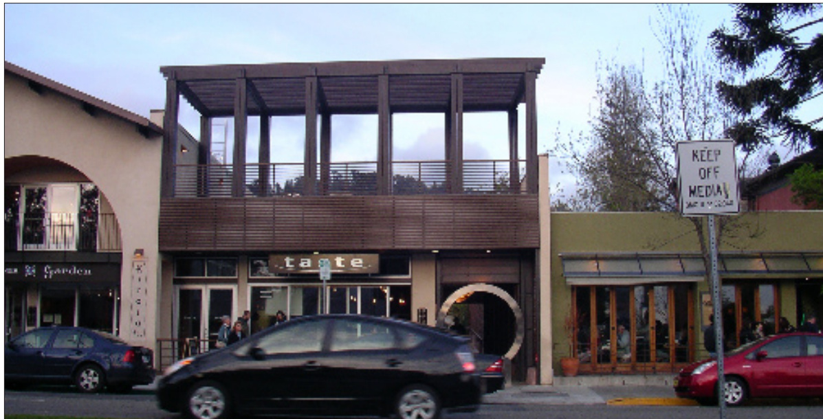
Second floor trellis treatment screening the mechanical equipment (1Avii-24)
