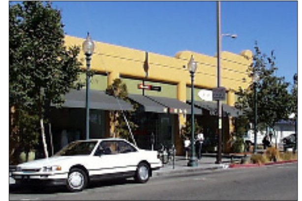
Signage mounted on awnings (1Ax-2)
