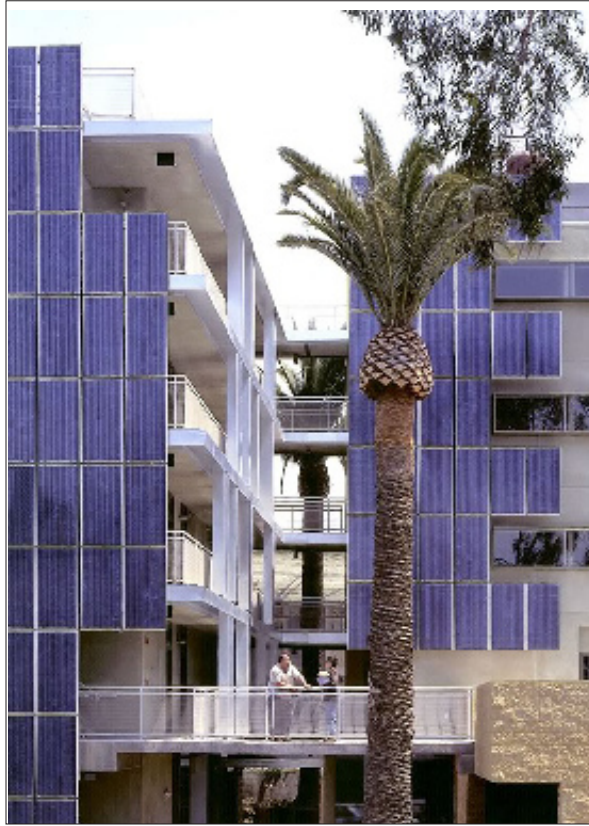
Solar panels as facade materials
