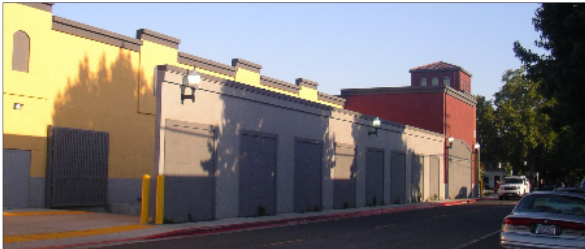
Service access of grocery stores (1Ci-2)
