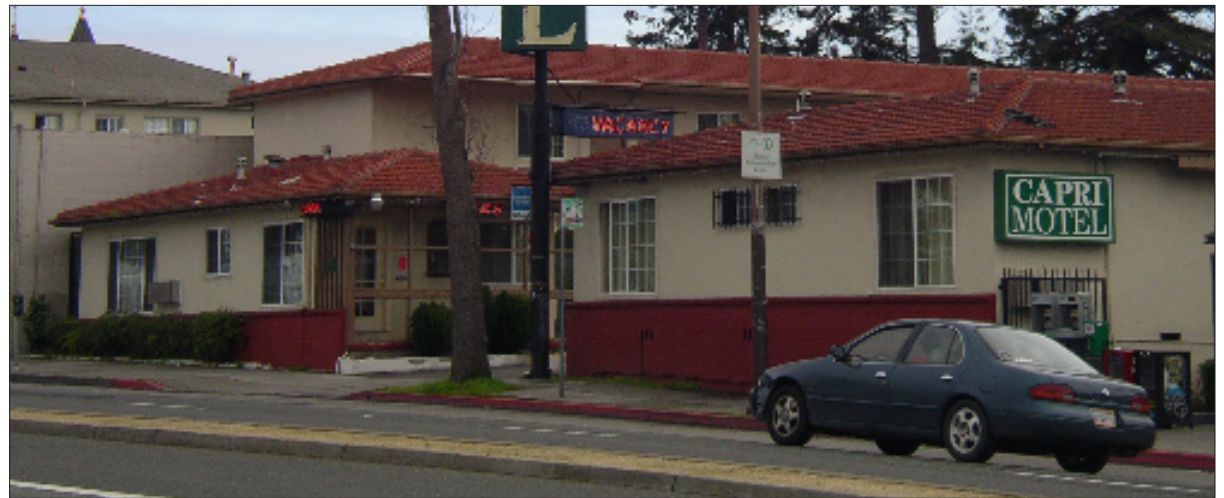
Pedestrian-friendly curb cuts
